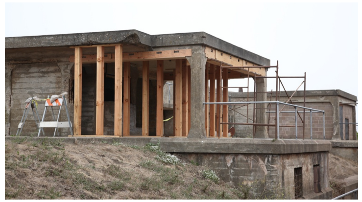
Concrete repair at Battery Godfrey, Presidio of San Francisco, 2012. Photo: National Park Service
