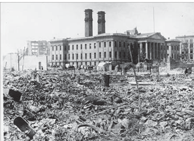
Old Mint after 1906 earthquake and fire (photographs courtesy of the National Archive Records Administration).
