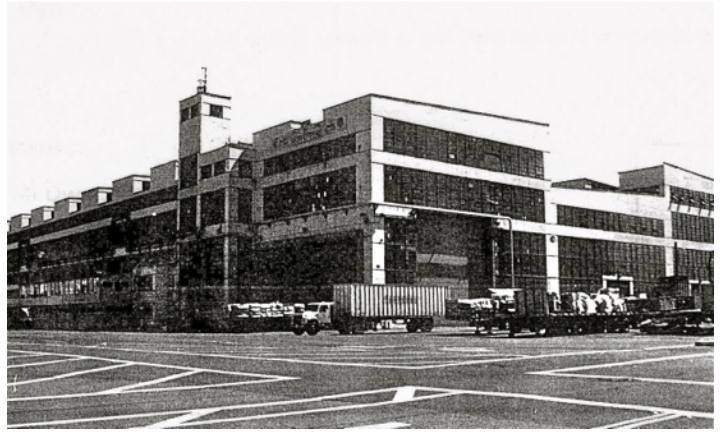
Building 386-388-390 (1922). Example of curtain wall construction, standard for industrial structures on Mare Island after World War I. Photo: National Register, Wes Gibson MINSY
